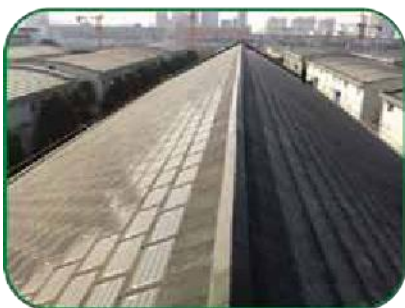
Install the counter batten and roof batten
