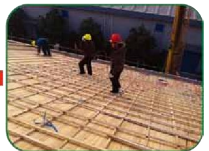
Cover the photovoltaic tile
