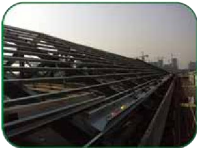
Build the steel bracket
