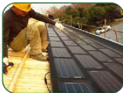
The photovoltaic tile roof is completed
